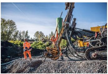
(3) A total of 140 micropiles are being installed on the individual foundations of the new bridge.
