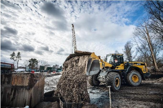
(3) A total of approximately 2,200 m<sup>3</sup> of polluted soil will be replaced and removed in special containers.
